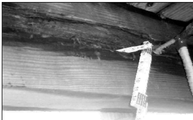
Exhibit IV. 1 Severely decayed timber beam
